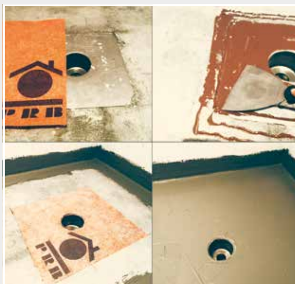
Platine inox + "Platine" en Natte Céramic.
