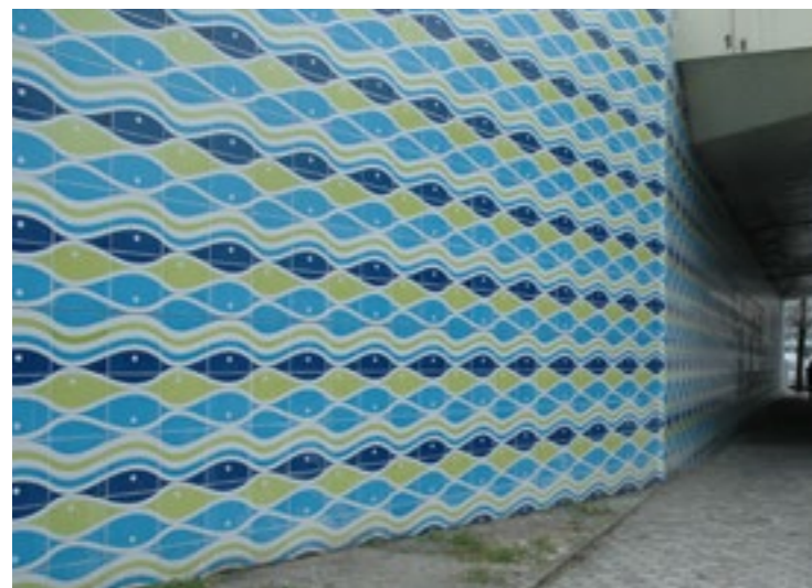
Túnel _ Aveiro, Portugal Tunnel _ Aveiro, Portugal
